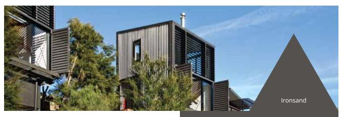
Each of the three component parts is clad and roofed with ColorCote® AlumiGard™ pre-painted aluminium. The Ironsand colour was chosen to fit with the marine environment.
